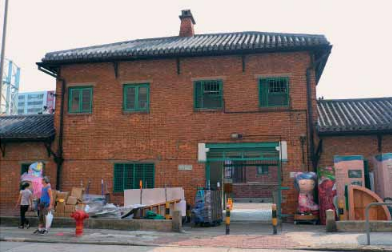
The entrance of the Cattle Depot. The workers are taking down the exhibition panels and the large doll called Fatina. They were part of the Hong Kong Heritage Tourism Expo (2010–11) of the Development Bureau. Photo: Celine Y. Lai.
