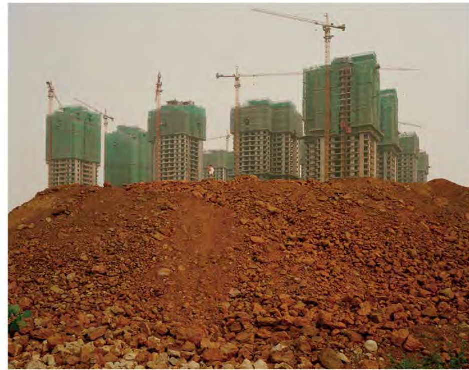
· Chongqing III, Chongqing Municipality, "Yangtze, The Long River"
